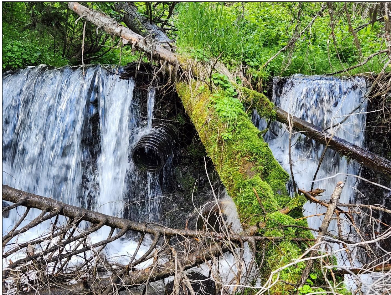
Figure 3. Gabion basket with corrugated plastic pipes in Squilchuck Creek.
